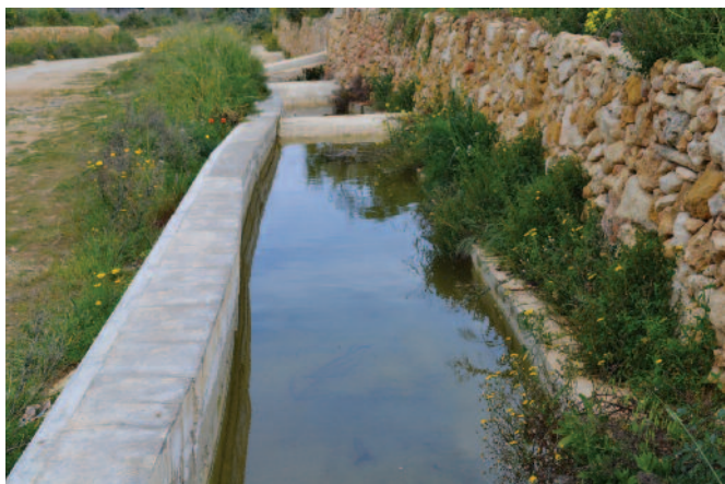
Figure 5. Roadside run-off is stored behind check dams for subsequent crop irrigation
