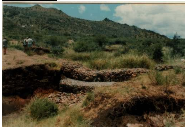
Gabion structures in gullies
