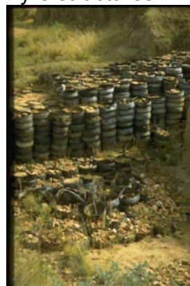
Tyre structures bound with wire and filled with stones
