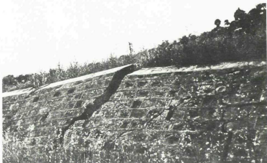
Plate 8. A concrete wall constructed over an earthflow along the road from Ain Draham to Fernana.
