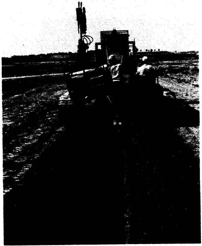
Fig.7.7: Installation of clay drains.
