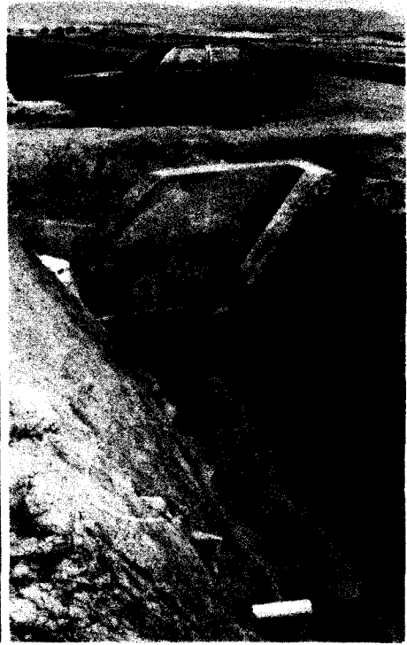
Fig.7.12: Concrete culvert below road.
