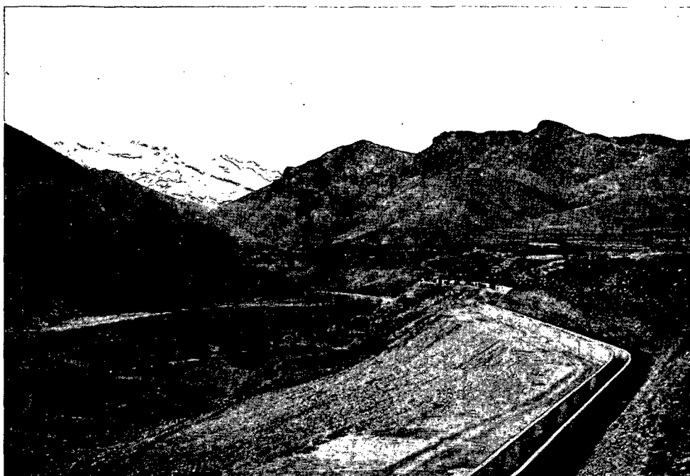
FIG. 134. A concrete flume is being constructed. It will carry water from a small dam, built in a tributary of the Lesser Zab in the mountain valley in the background. Deep Chestnut soils on the terraces of the Sungassar valley will be irrigated in the future.
