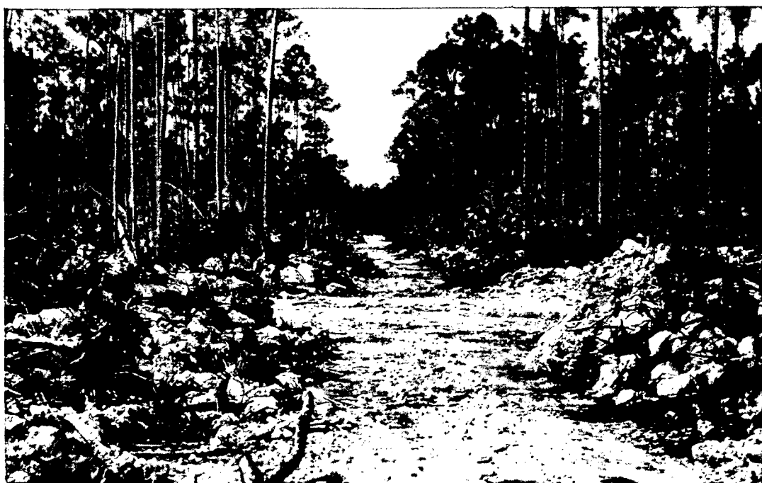
PLATE 4 Bulldozed third-order forest tracks prior to felling of the trees. Note the palmetto understory. The large blocks of limestone along the roadside, indicate land unsuitable for tillage; block 3a, North Andros.
