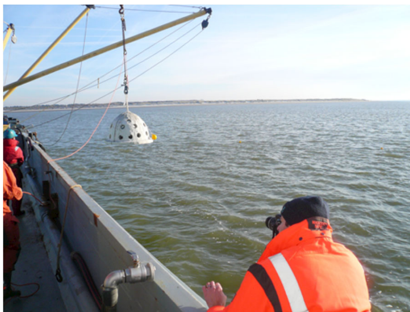
Figure 7. Reef dome being deployed at sea in the Voordelta.
