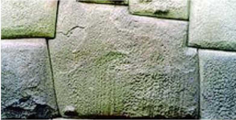
Construction of a wall in Cusco, using carved multi-angular stones and no mortar
