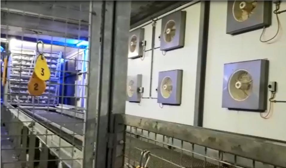
*Permanent fans along the side wall of a poultry lairage area in the Netherlands ©Storteboom*
