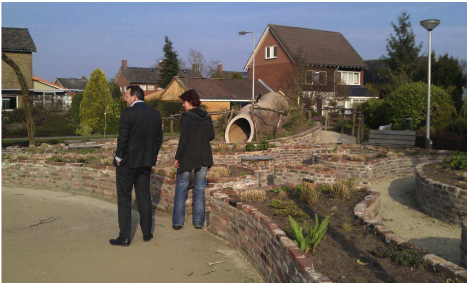
Fig. 2. DIOF under construction, April 2013.
