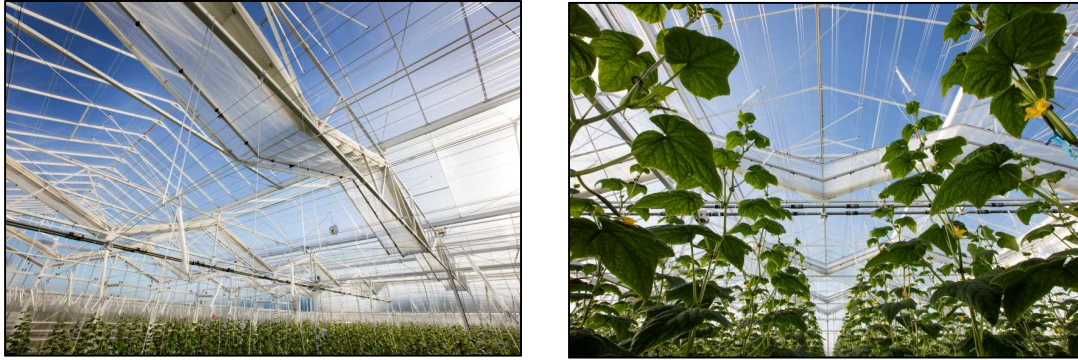
Figure 6. Photos of the final Winter light greenhouse with a partly closed W shaped double screen.
