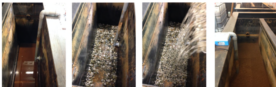
FIGURE 20: FILLING OF THE TANKS WITH GRAVEL AND IRON PELLETS
