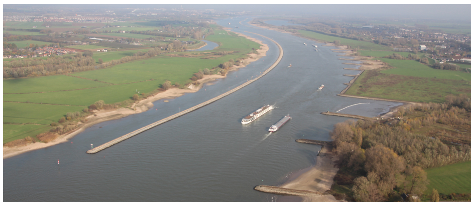
Figure 4.2: Longitudinal training wall replacing transverse groynes in the Waal River near Tiel. Source: Rijkswaterstaat.
