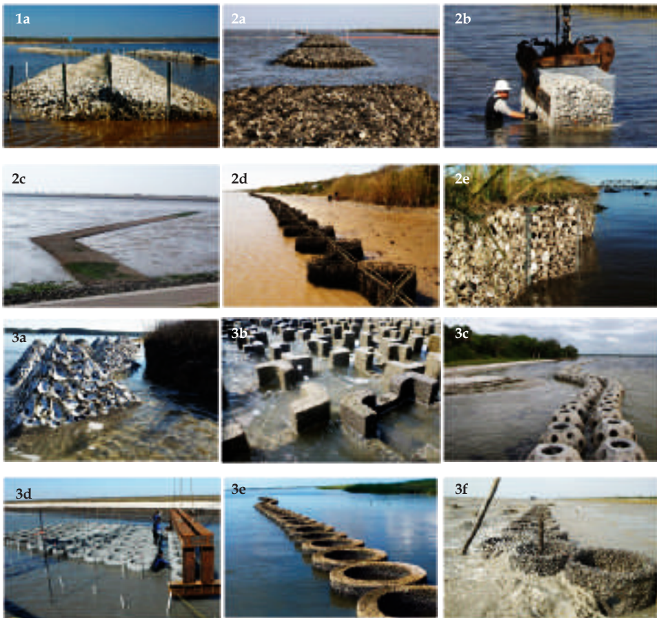
Fig. 7.2 Different eco-engineered oyster reefs used for coastal protection: (1) high-relief planted culch (1a. piles of oyster shells, Alabama, USA); (2) contained culch (2a. shells on mesh bags, Alabama, USA; 2b. Shell in gabion boxes, Louisiana, USA; 2c. Oyster shell covered by gabion mesh, Oosterschelde, The Netherlands; 2d. Reefblk, Louisiana, USA; 2e. HESCO delta unit, Louisiana, USA); (3) Precast concretes (3a. Concrete pyramid having oyster shell on surface, Virginia, USA; 3b. Oyster castle or tower, Virginia, USA; 3c. Reef balls, Florida, USA; 3d & 3e. OysterBreak, Louisiana, USA; 3f. Breakwater oyster reefs (Kutubdia Island, Bangladesh). [Photos were taken from different internet sources such as TNC, BwN, CHE, etc.]
