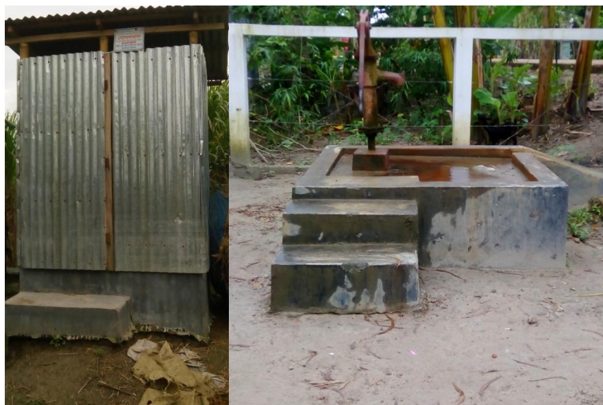
Photo: The toilet and tubewells are put at a higher than the grounds level to safe the structure from damage from flood water in the NGO intervention area. These are made with the support of NGOs. Source: Researcher.
