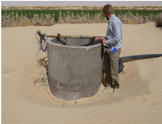
Fig. 28. A simple well to supply water to the pivots
