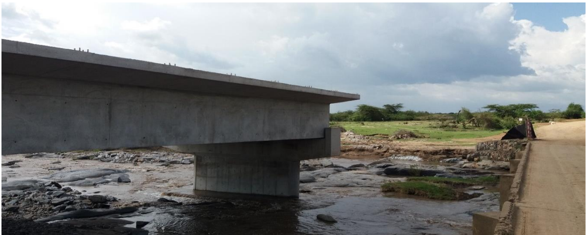
Figure 13: Ongoing construction of a bridge in the Mara
