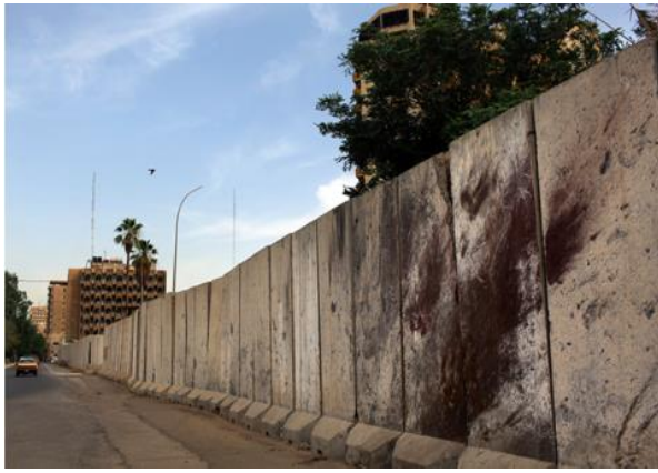
Figure 3: Concrete Blast Walls at Green Zone (Source: The New York Times , 2010b).
