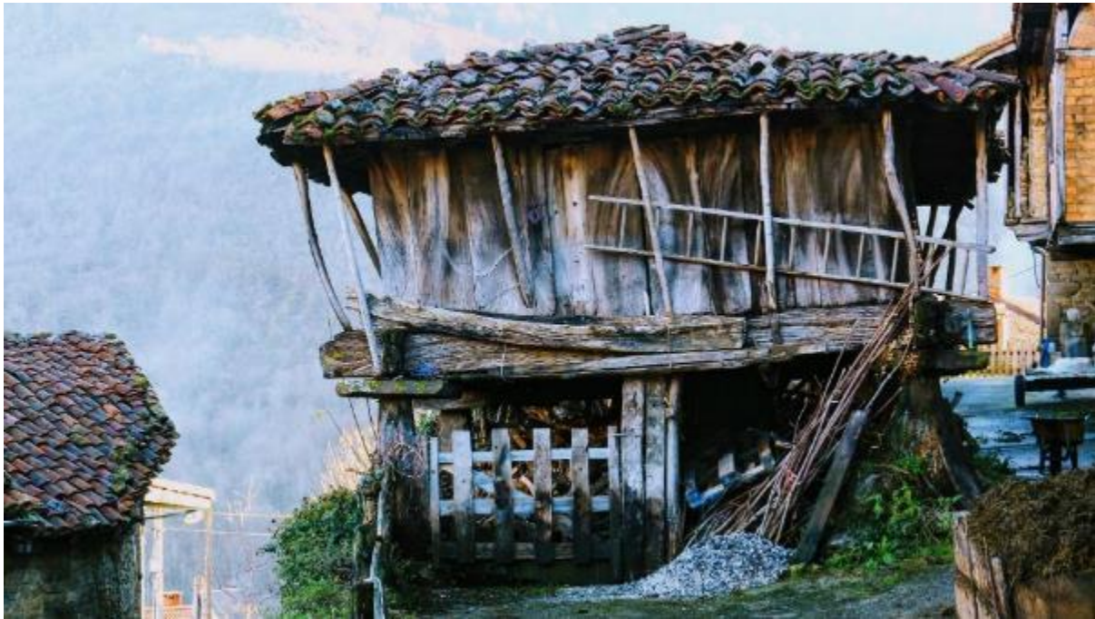
Image 5. A typical hórreo, a granary upon pillars to prevent the access of rodents. Source: Isabeau Ottolini
