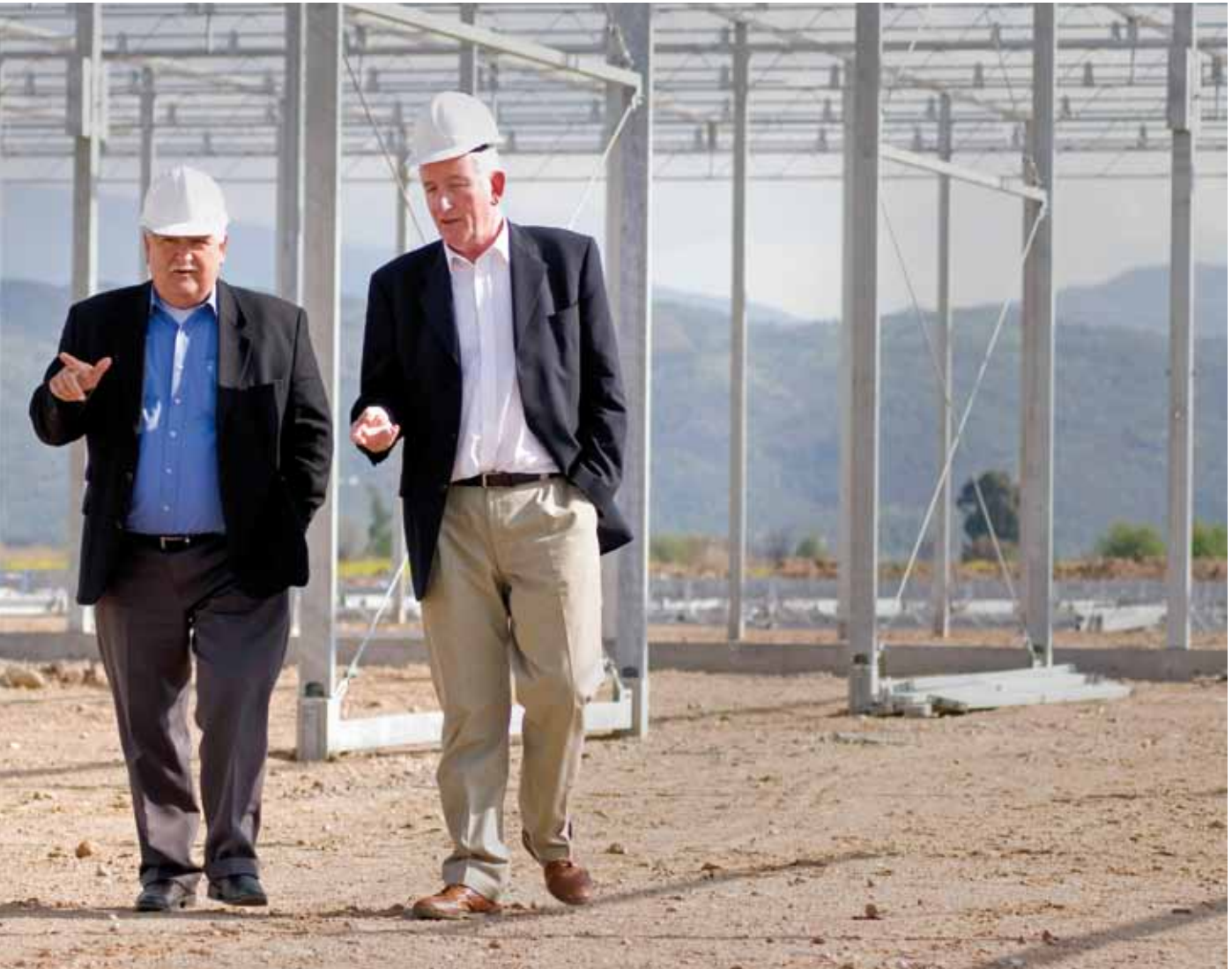
Ton Schrover and Ruud Maaswinkel in front of the skeleton of the new demonstration greenhouse.
