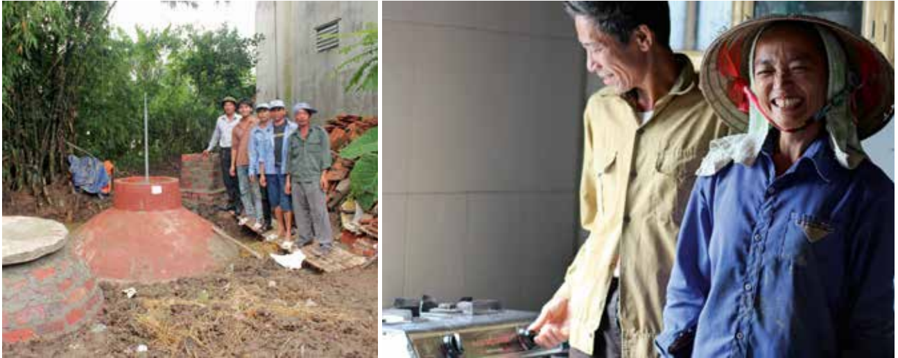
A new anaerobic digester is ready in Vietnam. The methane gas released will be used for cooking.
