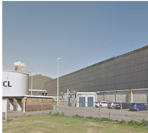
Pipelines (gas receiving station)
