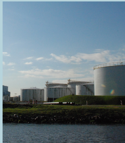
Fuel storage in Westpoort
