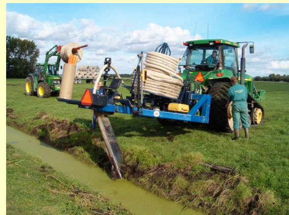
Installing the submerged drains below ditchwater level
