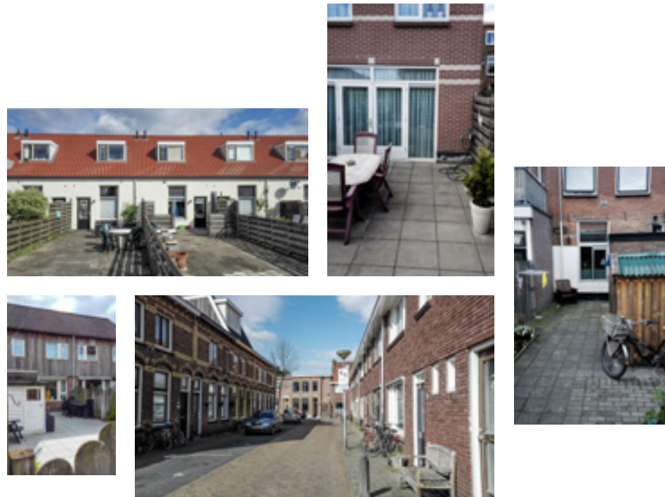
Figure 12-16. Many paved surfaces in the streets and backyards of Assendorp
