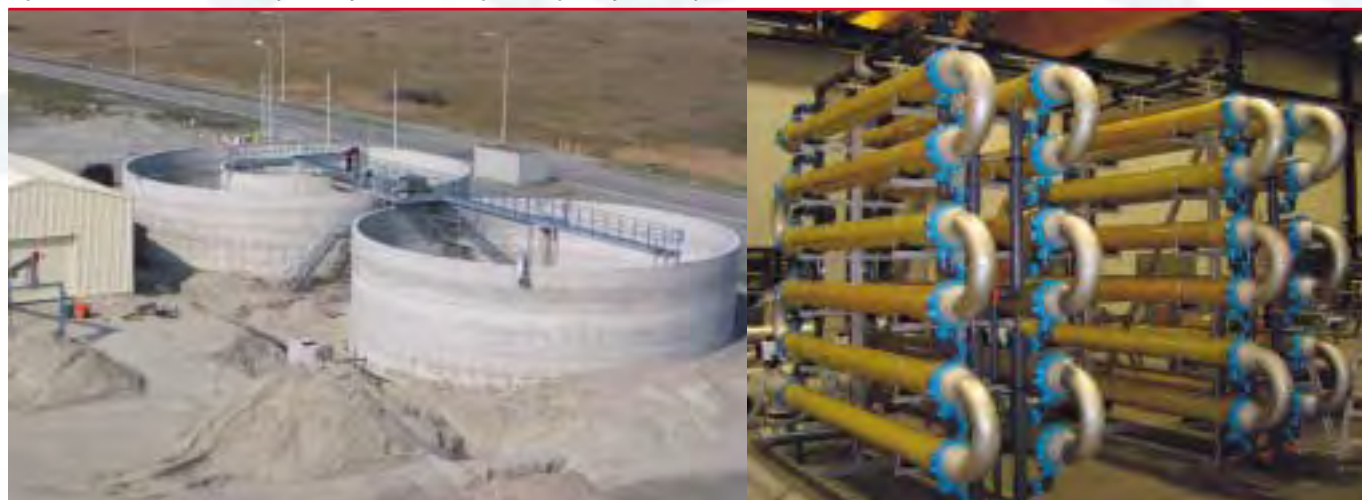
Figure 2: Membrane bioreactor system: (left) bioreactor; (right) 4-stage ultrafiltration system.
