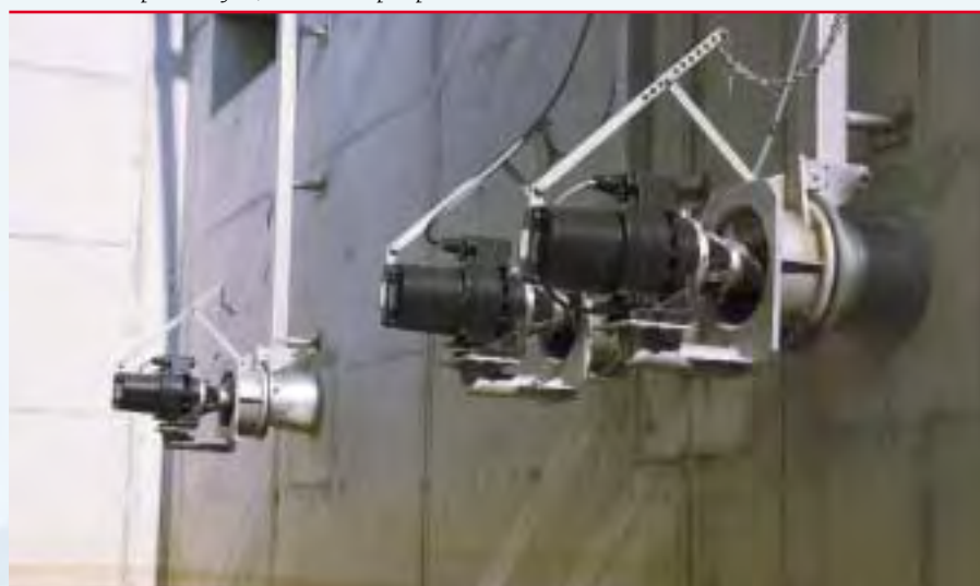
Membrane compartment feed/recirculation pumps.
