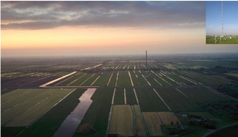
Figure 6. The 213-metre meteorological tower at Cabauw, the main platform of the CESAR consortium ( http://www.cesar-observatory.nl/ ). It is located between the cities of Utrecht and Gouda, in the Western part of the Netherlands (51.971° N, 4.927° E) in a polder region covered by grass and 0.7 metre above sea level. In addition to a complete set of meteorological and atmospheric composition observations at the tower and in the nearby surface, there are instruments using remote-sensing techniques like rain radar, and ceilometers. Courtesy and credit: Bert Heusinkveld.
