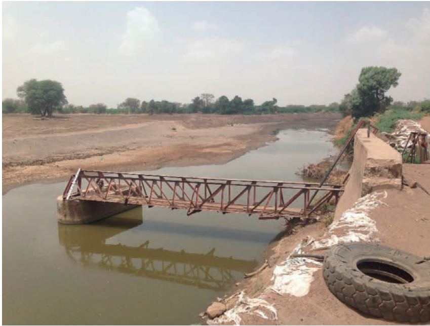
Figure 2 A large irrigation scheme near Metahara diverts a huge chunk of the river flow to irrigate thousands of hectares of sugarcane.
