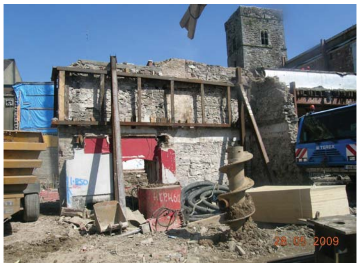
Figure 5.7: Braced portion of the upstanding town wall in advance of conservation works at Barronstrand Street, Waterford in advance of redevelopment of Penny's shop (© Margaret Keane).
