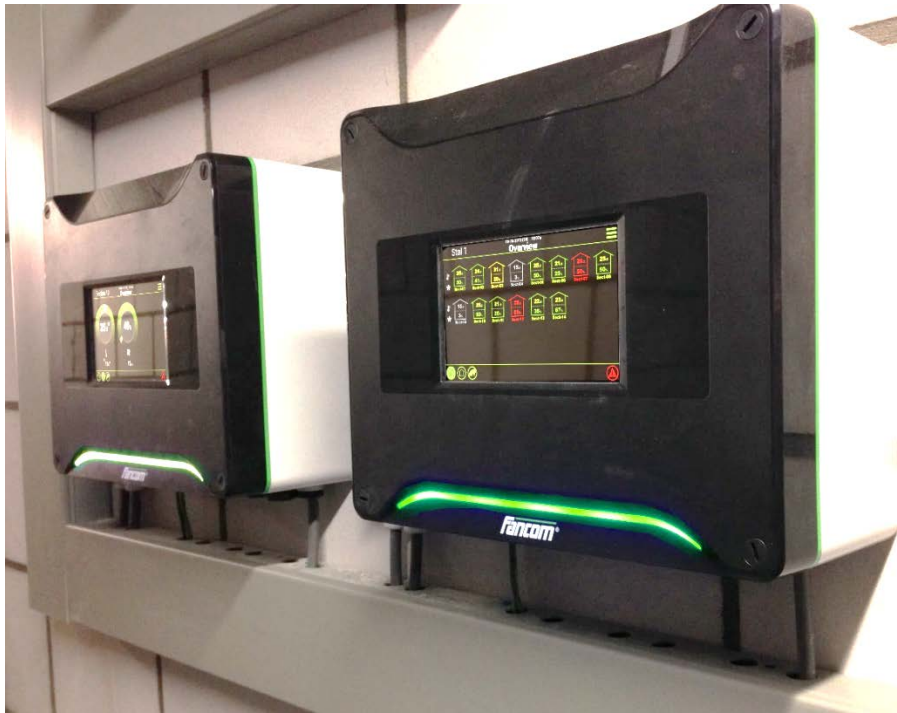
Figure 3.5 Climate control devices. Photo courtesy of Fancom
