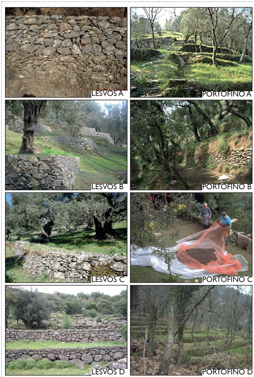
Figure 26: Pictures of terraces from Lesvos and Portofino: Lesvos A: Mixed masonry of schist with later limestone addition near Mytilini; Lesvos B: Olive nets on very well preserved individual limestone terraces near Agiassos; Lesvos C: Braided limestone terraces near Mytilini; Lesvos D: braided terraces with volcanic material near Kalloni; Portofino A: Embankments with olive yards; Portofino B: Supporting dry stone wall in undefined bond using blocks and elements from weathered conglomerate; Portofino C: Olive harvest at a small farmstead near Nozarego; Portofino D: Gentle terraced slope with low embankments, material originating from marl-limestone rock types.
