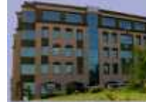
EEA Head Office Building
