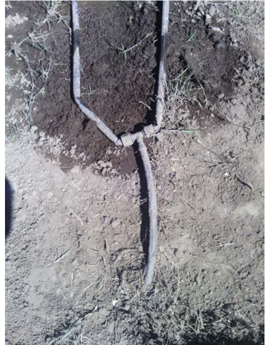
Figure 2- Typical repair for a broken lateral
