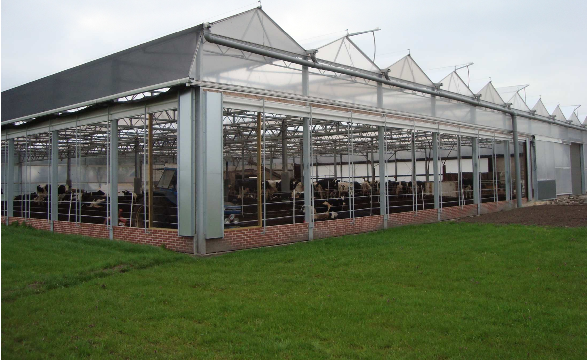
Roof from horticulture
