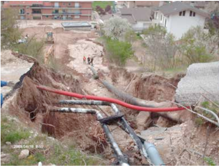
Figure 3.2.1. Damaged lifelines in l'Aquila 2009
