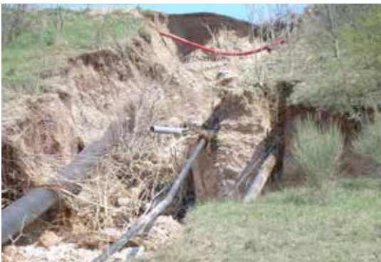
Figure 3.2.2. One of the main damages in 2009: Gran Sasso Aqueduct
