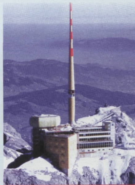
Säntis mountain station
