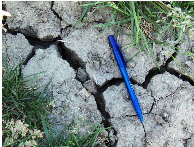
Fig. 1.1 Shrinkage cracks in a clay soil. Pen for scale.
