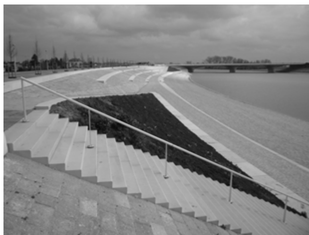
Figure 4. New quayside along the newly created 2 km long side channel in the River Waal near Nijmegen and Lent (photo: J.M. van Loon-Steensma).
