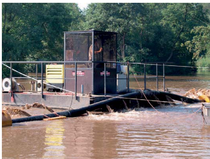
Fig. 4.6: Application of sand capping in Lake Kleine Melanen (7 September 2012).
