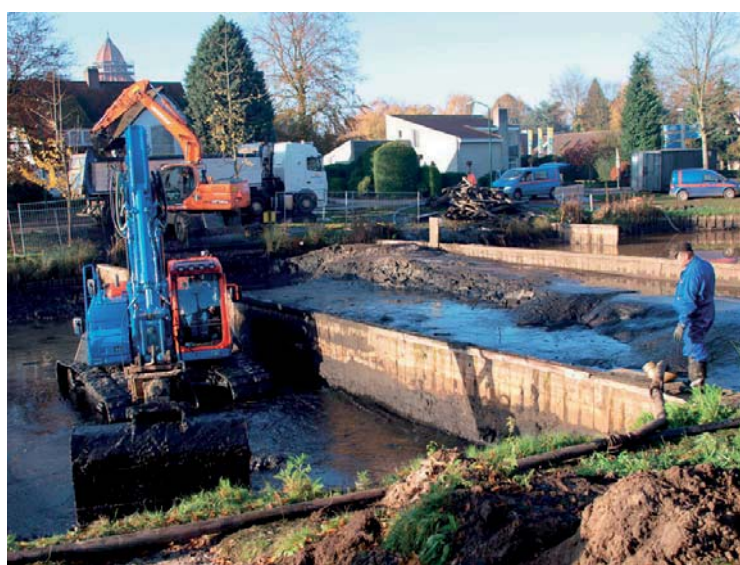
Fig. 3.3: Sediment removal at pond Dongen (10 November 2011).
