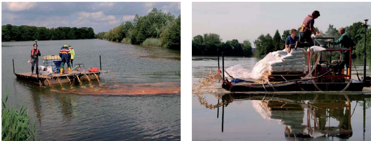
Fig. 5.3: Application of iron(III)chloride (18 May 2009, left panel) and lanthanum-modified bentonite (LMB, 19 May 2009, right panel) at Lake De Kuil.
