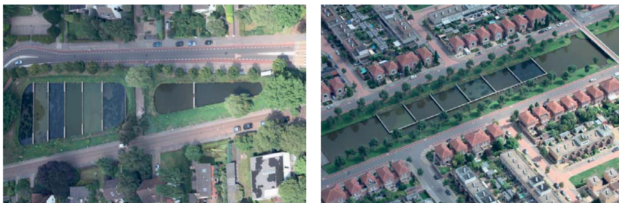
Fig. 3.2: Aerial view of the compartments at pond Dongen (left panel) and pond Eindhoven (right panel). Photographs by L. Turlings, 11 August 2010.
