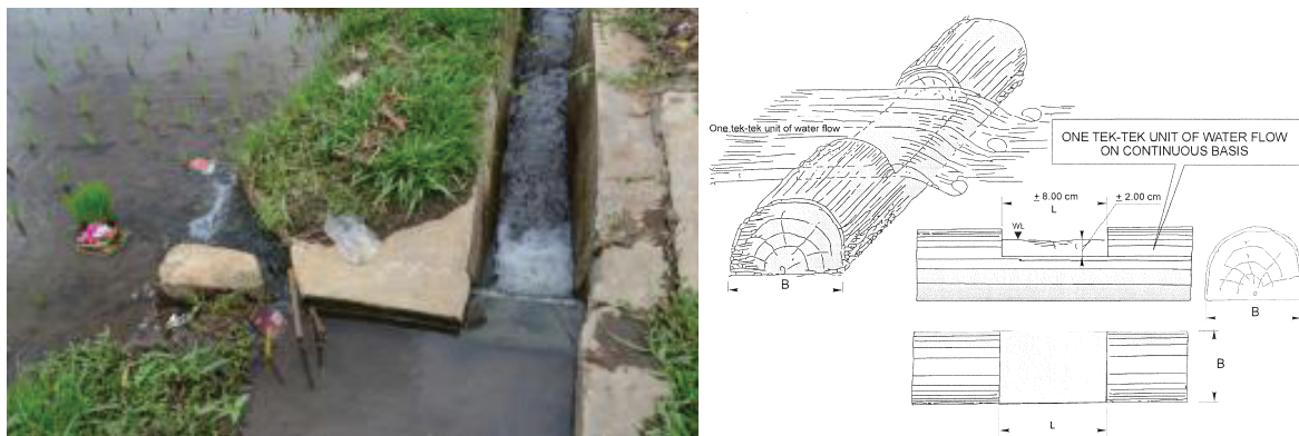
Figure 3.4. Typical water distribution unit ( tektek or kecoran )
