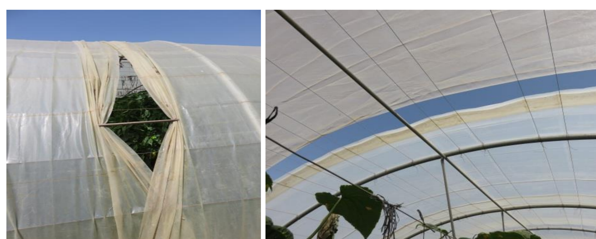
Figure 2: Tunnel with (too) small opening to ventilate (left); right a reasonable good ventilation slit
