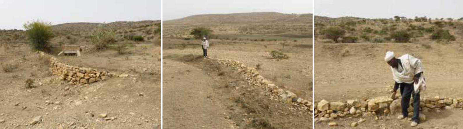
Farmers have built stone bunds to divert water from roads to their farms. Photo: MetaMeta
