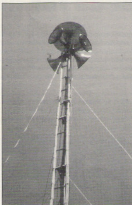
The CATS consists of a karaoke system (an integrated sound unit with double cassette player, very popular for entertainment in Asia), two microphones, an amplifier with a 500 watt power output capacity connected to four 100-watt loudspeaker systems attached to a metal pole. Total cost: US$ 2,000 approximately. These are housed either in a specially renovated room in the barangay centre or in another place agreed upon by the community. "Broadcasts" can reach up to a two-kilometre radius so that in some sites, other adjoining barangays benefit as well from the information dissemination.
