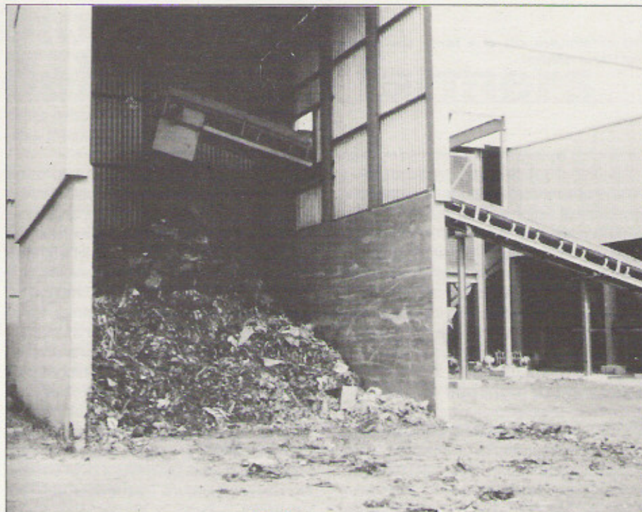
Photo: WASTE Consultants
