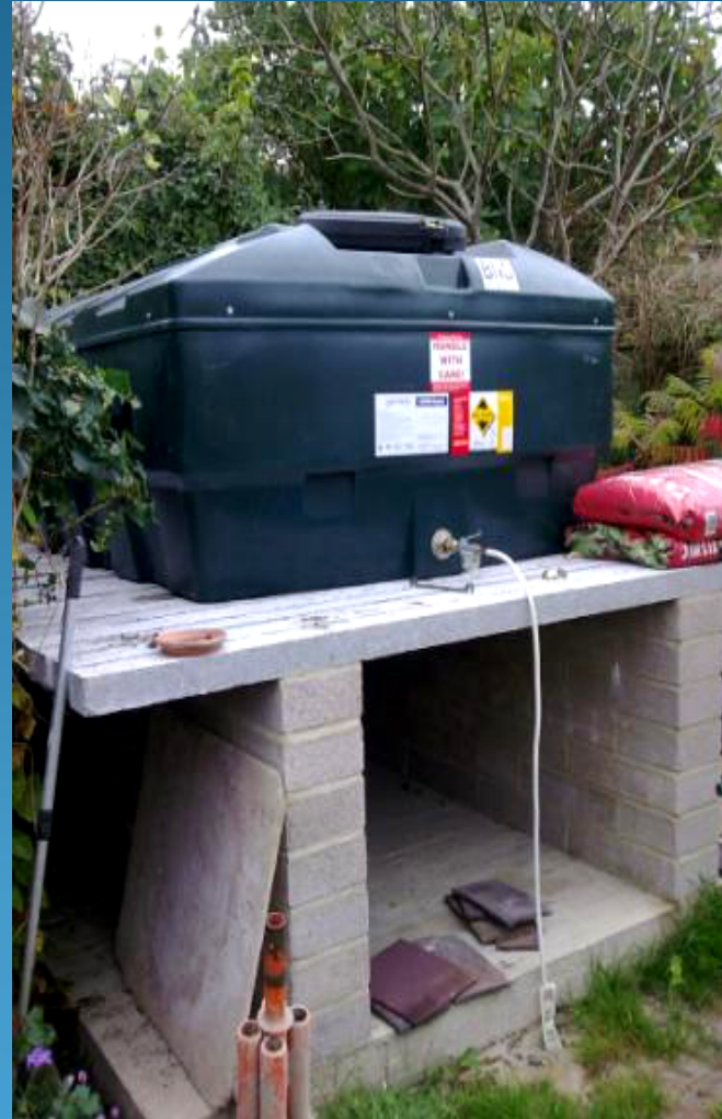
Oil tank above flood height
