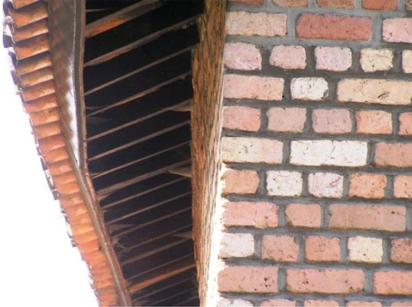
*Figure: The outer wall of the classroom forced out by the roof beams*
