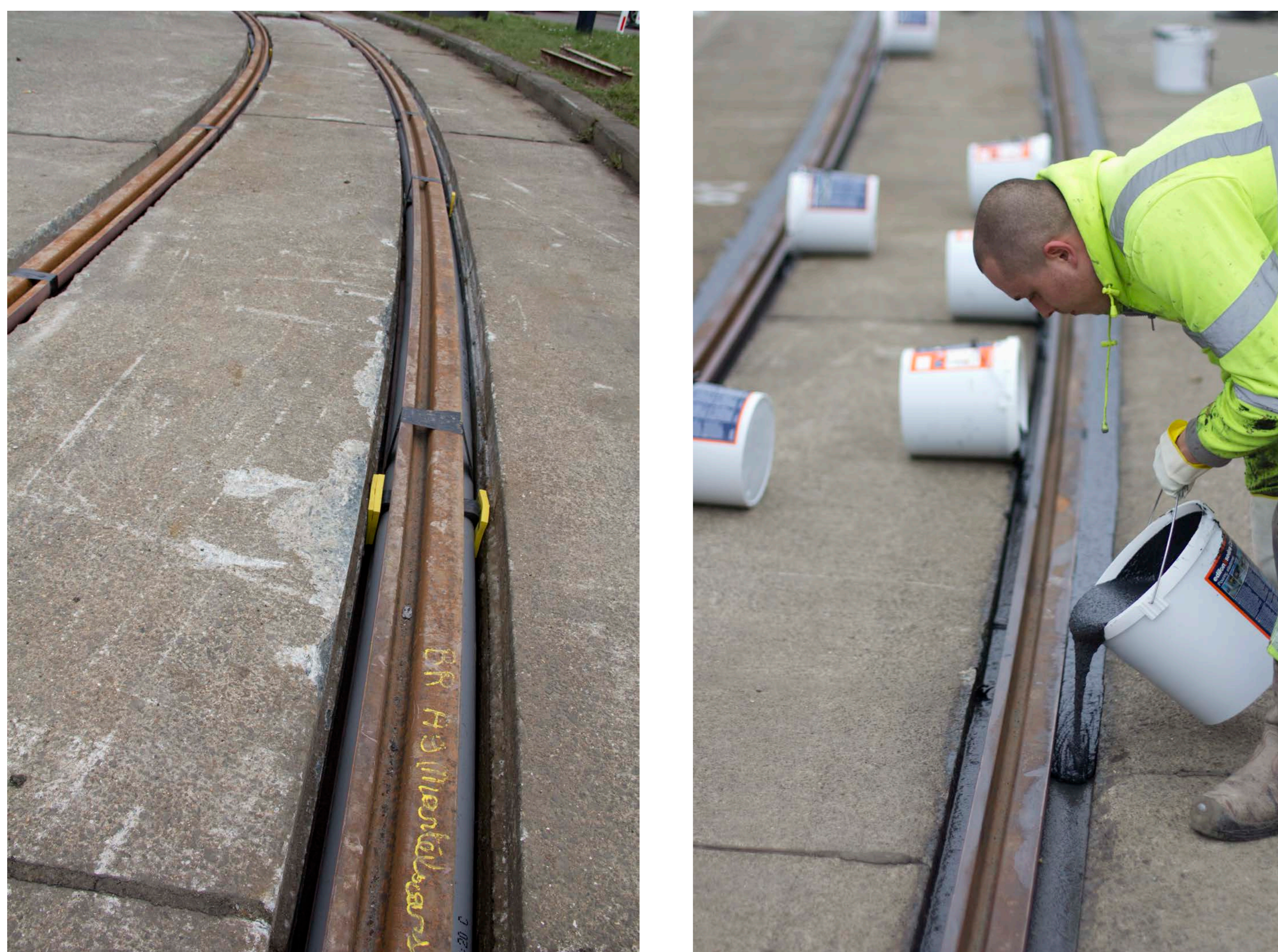
Figure 1. Example of a sustainable edilon)(sedra product application, reducing rail wear in curved tracks.
