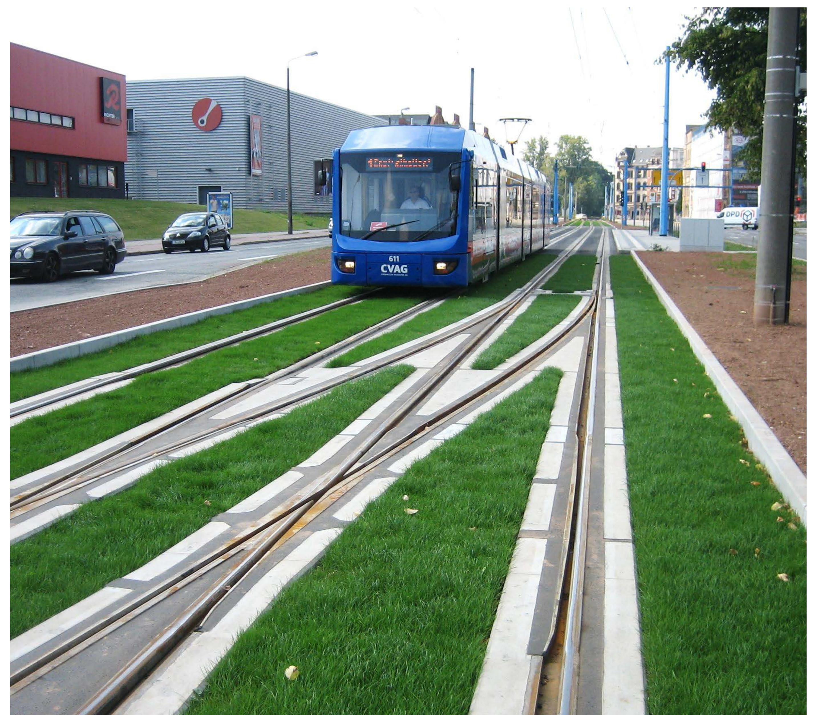
Figure 2. Example of a rail track embedded in noise & vibration dampening elastomer.
