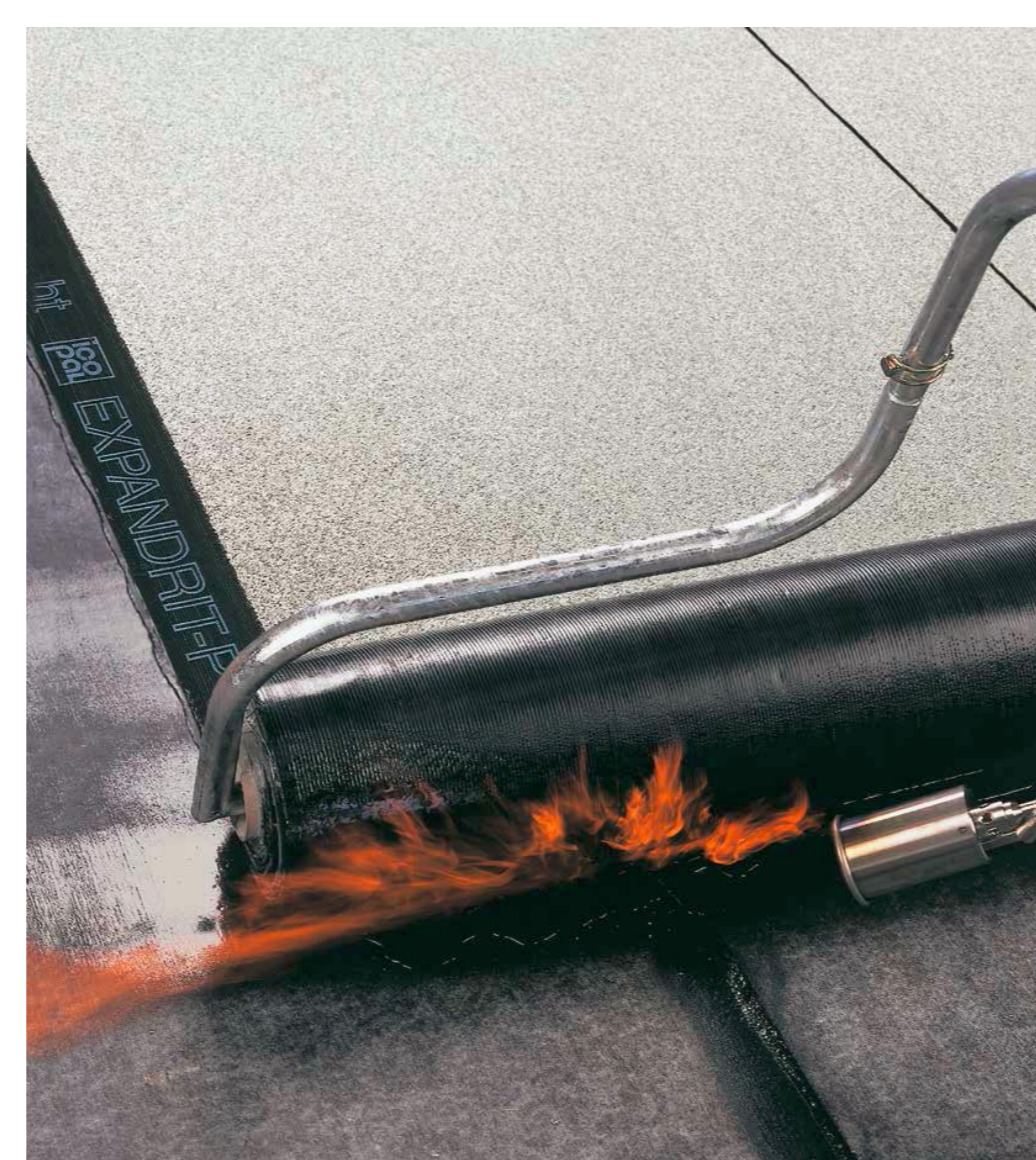
Figure 2. Installation of a bituminous roofing membrane
