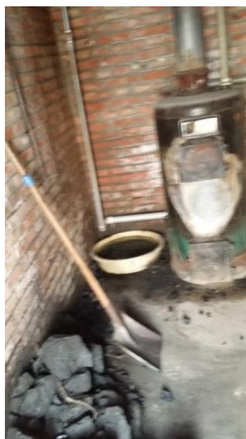
Figure 7.7. The boiler for green house heating
