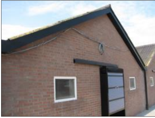
Inlet opening (outside the room)
