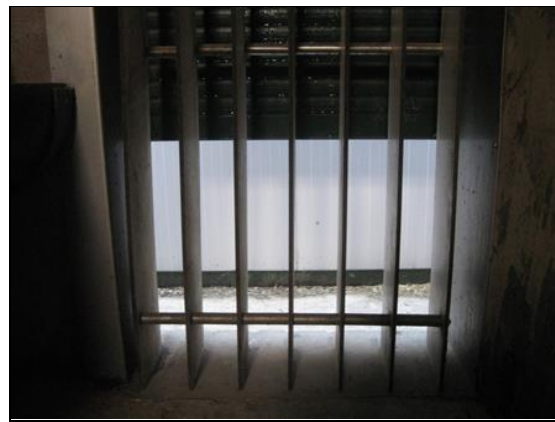
Inlet opening (inside the room)
