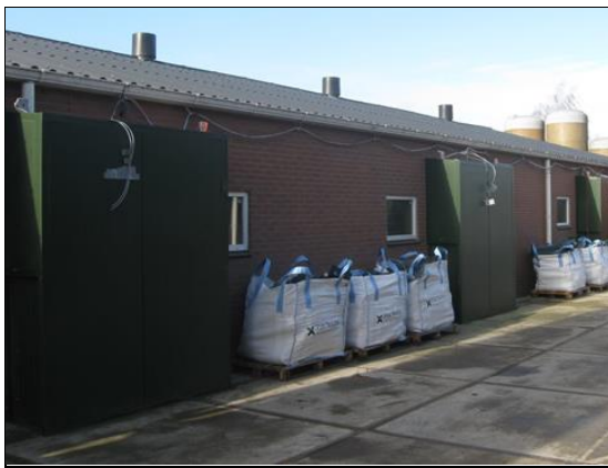
Inlet opening (outside the room)
