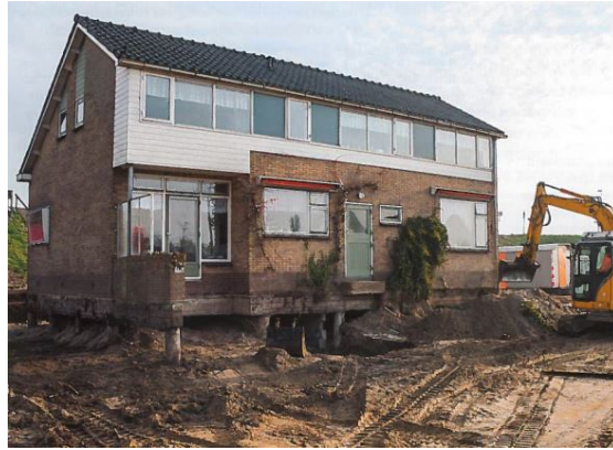
FIGURE A.2: Preparation of jacking up a building near the Lek dike (van Leeuwen and van der Giessen, 2015)
